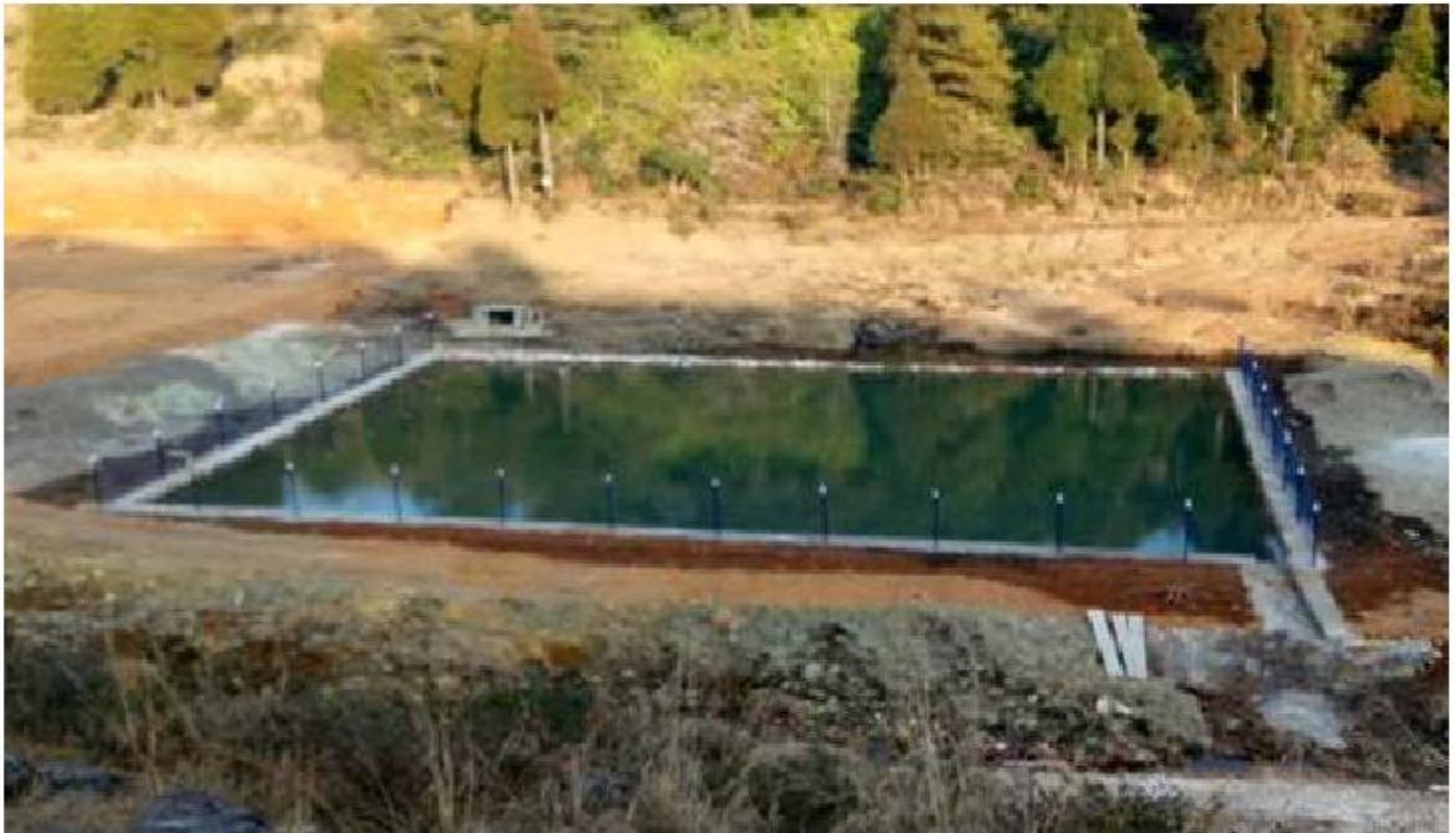
Newly constructed Rain water harvesting East Khasi Hills, Meghalaya
